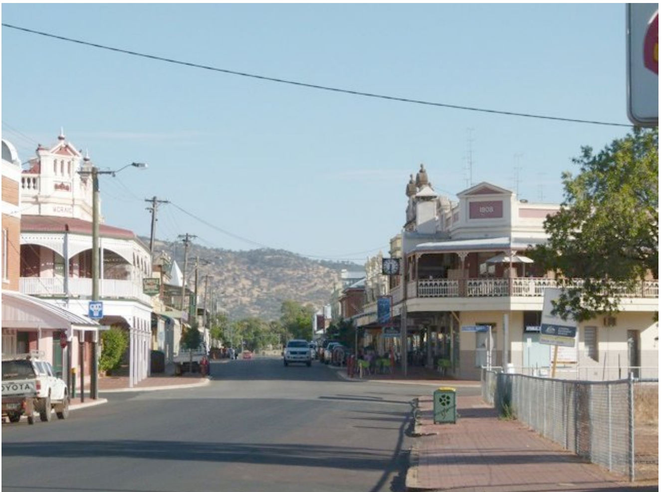
Avon Terrace looking north 2014
