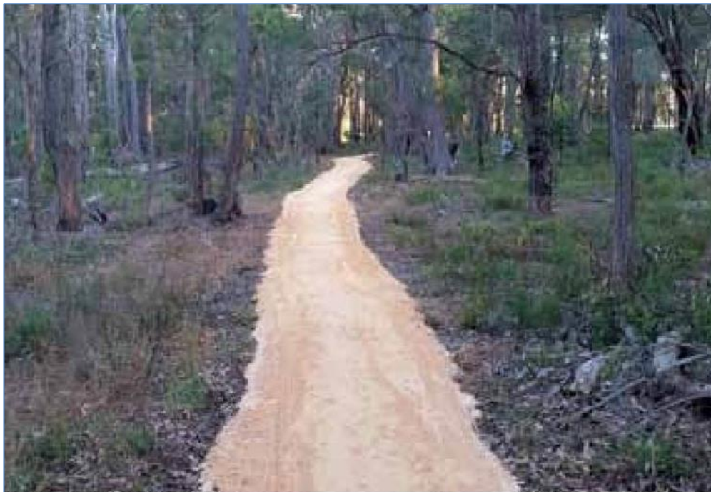
Photo 10: A 'green bridge' of limestone through a Dieback infested area on a track (source: Kaylene Watts).
