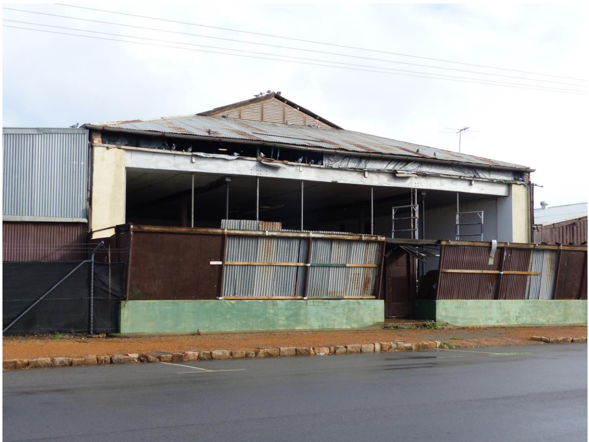
Derelict building C Clarke 2017
