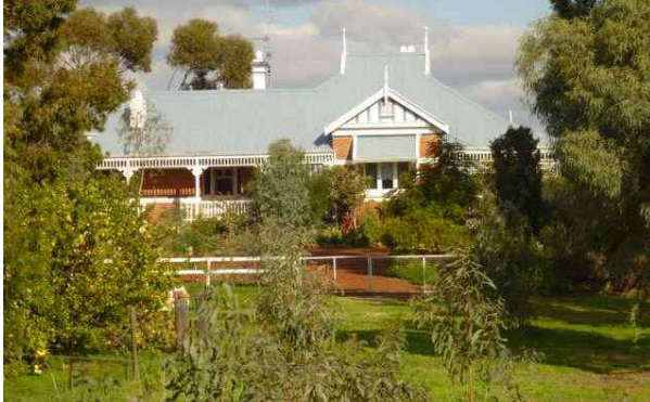
View from Fraser Street
