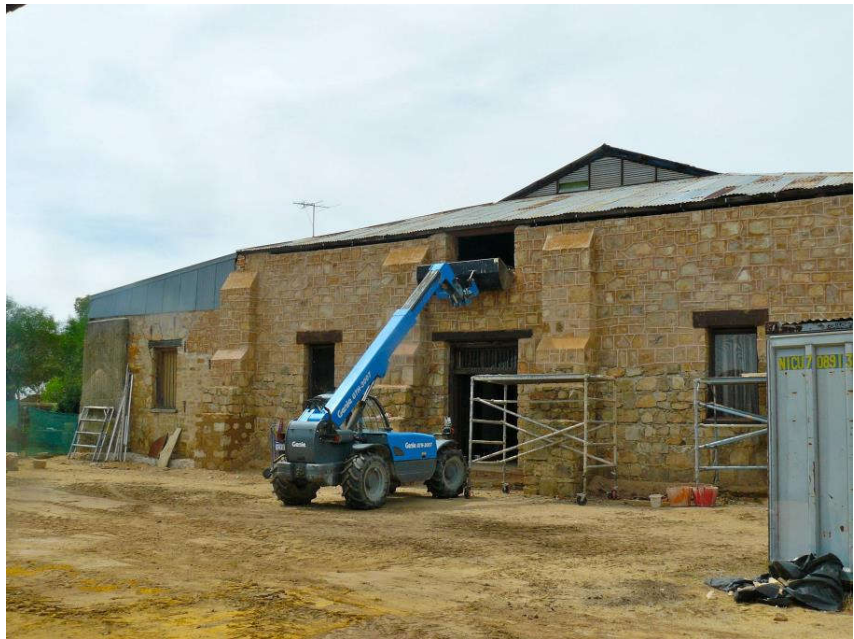
Rear wall restoration 2011
