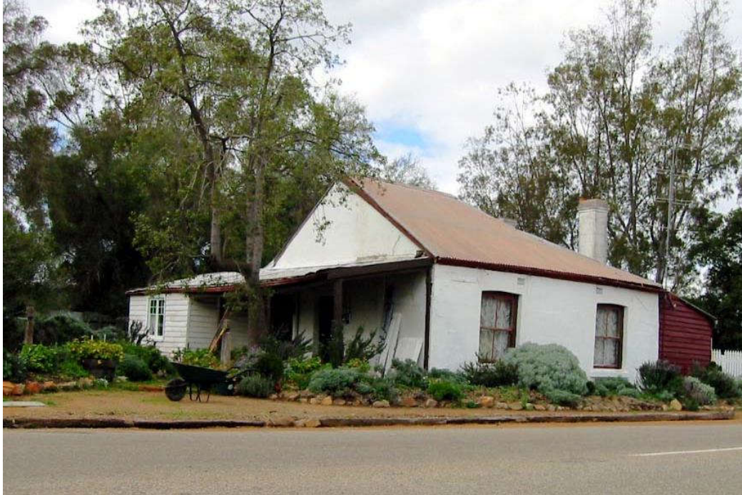
c.2004 Photograph (Gable facing Redmile Road)
