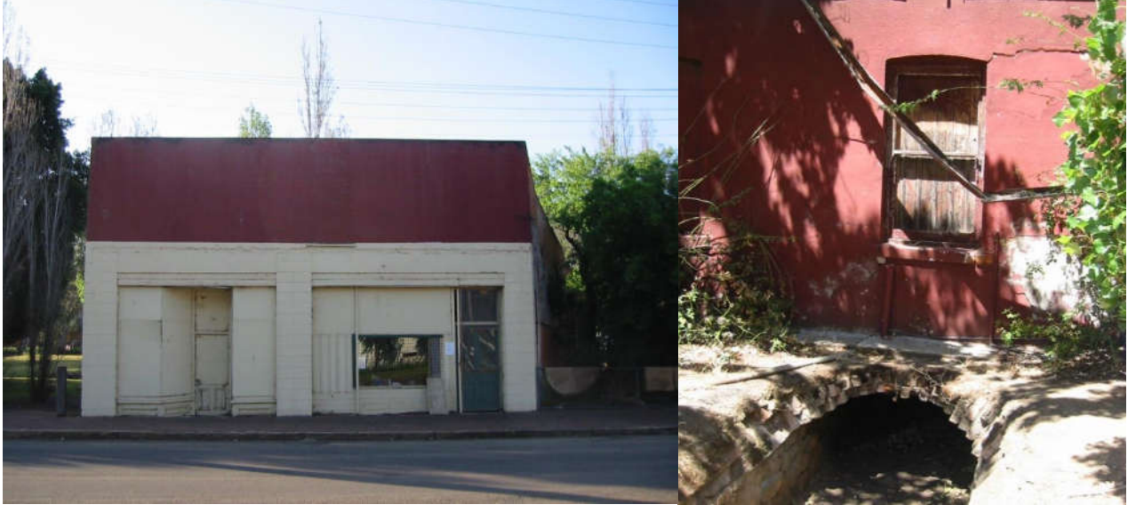
Photos: 2004 prior to demolition in 2005.
