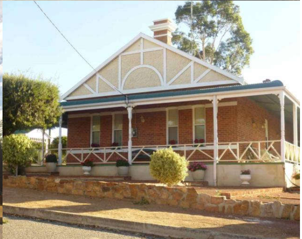
Alfred Street frontage
