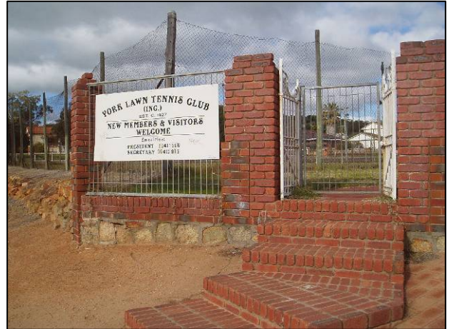
Entrance to club – steps and steep ramp
