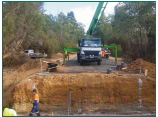
Talbot Road West Bridge Replacement
