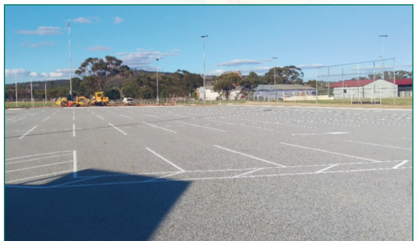
York Recreation and Convention Centre Carpark
