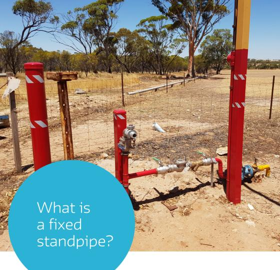
A fixed standpipe is a metered service which provides access to bulk water supplies directly from a point on a water supply main.
