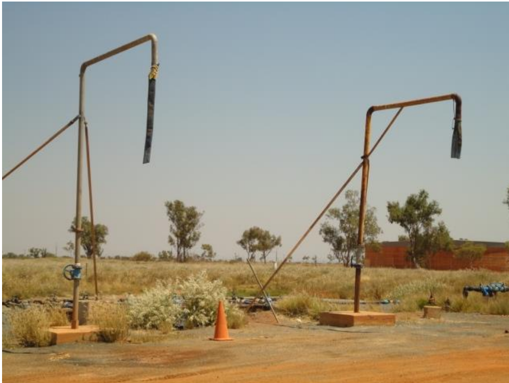
Figure 2: Standpipes that the above meters are feed to
