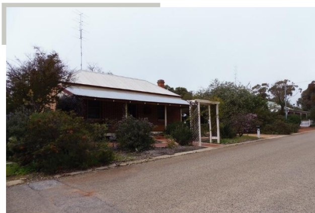
12 Thorne Street, York Source: SCA 2020
