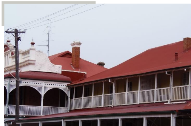
Castle Hotel & Outbuildings 95 -97 Avon Terrace, York Source: SCA 2020
