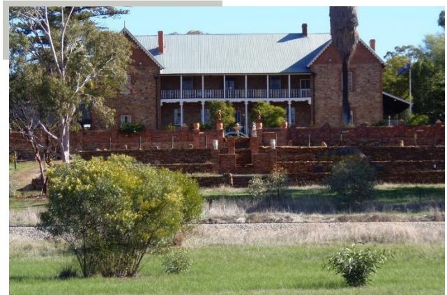
Faversham House Source: SCA June 2020
