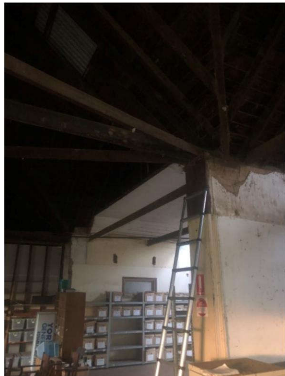
Three splayed Timber Members across the Front Room
