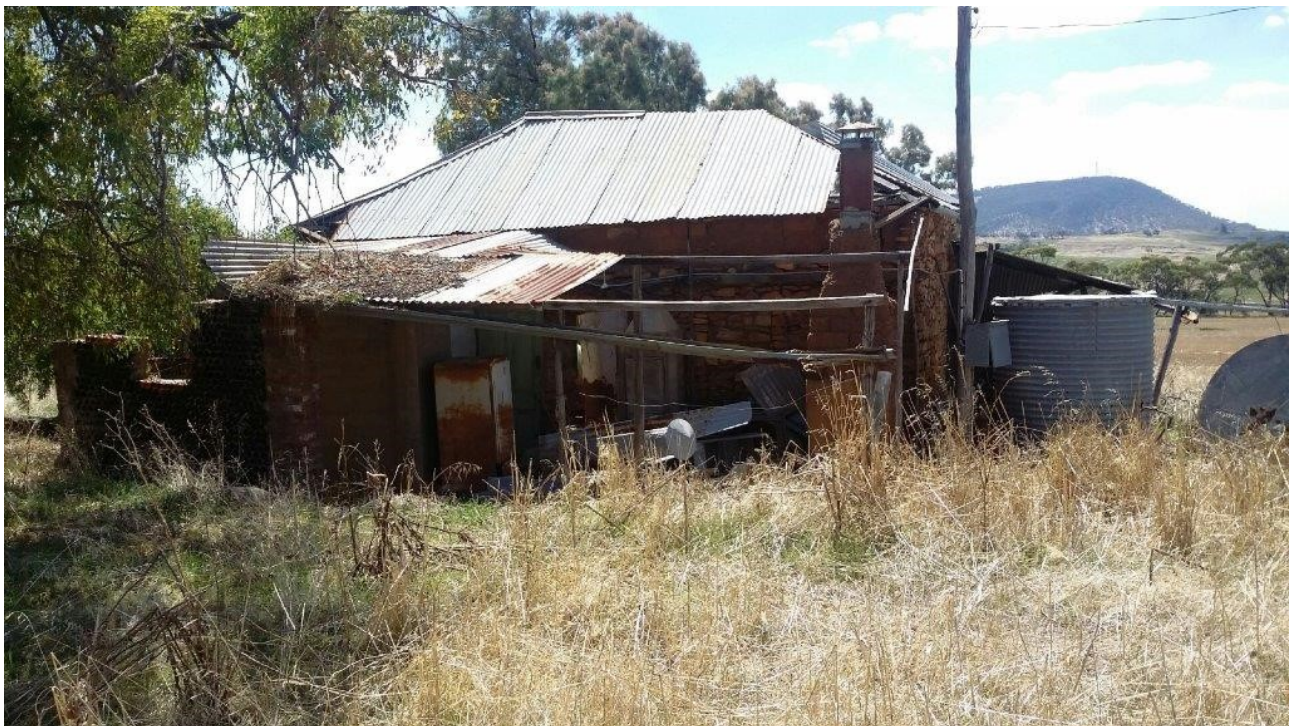
“Fairview” Ashworth Road York. Now an abandoned homestead.
