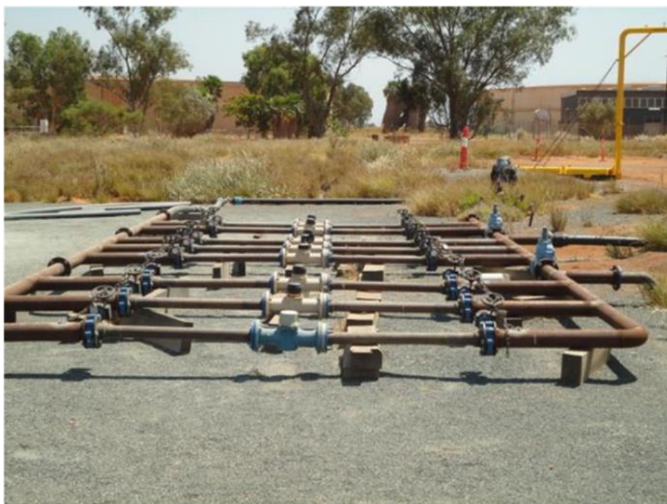
Figure 1: Eight lockable WC meters supplying two standpipes (see Figure 2) that customers access under a Special Agreement
