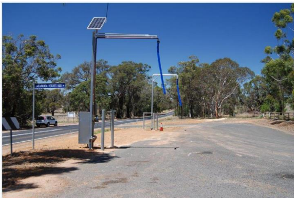
Figure 6: A card operated standpipe that dispenses potable water, the 2nd standpipe supplies non-potable water, both standpipes belonging to Kojonup Shire
