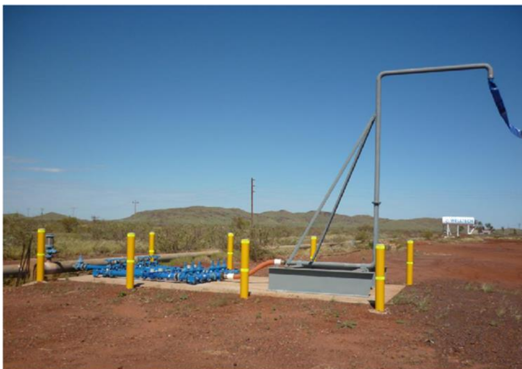
Figure 3: A bank of 6 meters, each with separate locks that can be access by customer under the terms of a Special Agreement.
