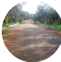
Construction Clearing culverts and drains
