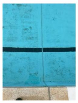
Cracking in the pool floor
