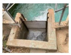
Broken strainer screen (Balance Tank)
