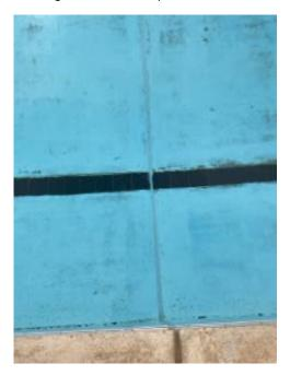
Different width of the expansion joint sealant
