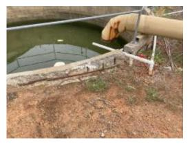
Spalled concrete wall and rusted reinforcement
