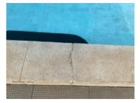
Concrete upstand cracking (no handrail)
