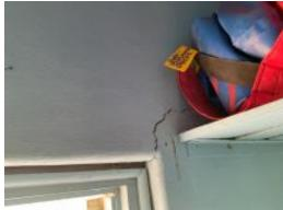
Structural crack above Plant Room door
