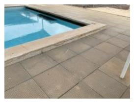
Concrete upstand cracking
