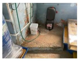
Degradated concrete plinth and brick wall
