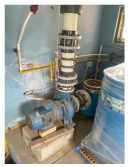
Insufficient pump fixing
