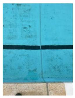
Cracking in the pool floor
