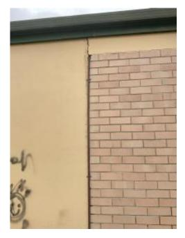
Separation between Filter Tank and Plant Room
