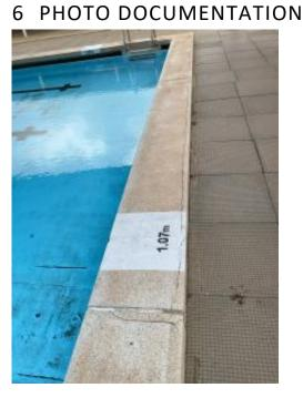
Cracking in the concrete upstand
