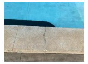
Concrete upstand cracking (no handrail)
