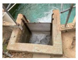
Broken strainer screen (Balance Tank)
