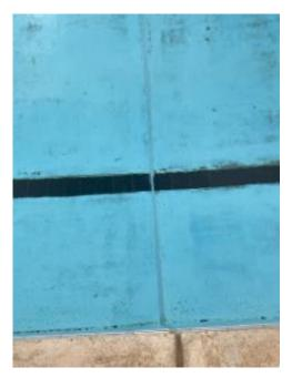
Different width of the expansion joint sealant
