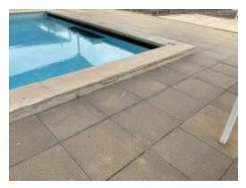
Concrete upstand cracking
