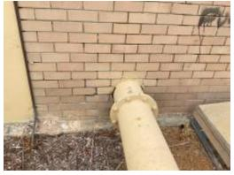
Damaged mortar around the pipe
