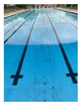
Cracking along centre line
