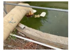
Damaged Balance Tank wall, rusted pipe and rubbish
