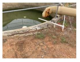
Spalled concrete wall and rusted reinforcement
