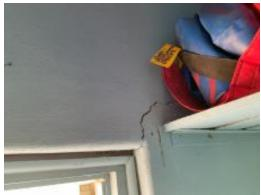
Structural crack above Plant Room door
