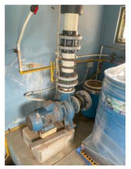
Insufficient pump fixing
