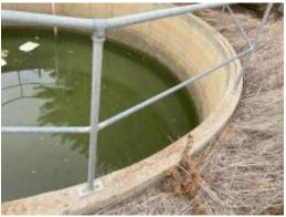
Cracked wall and unsafe balustrade
