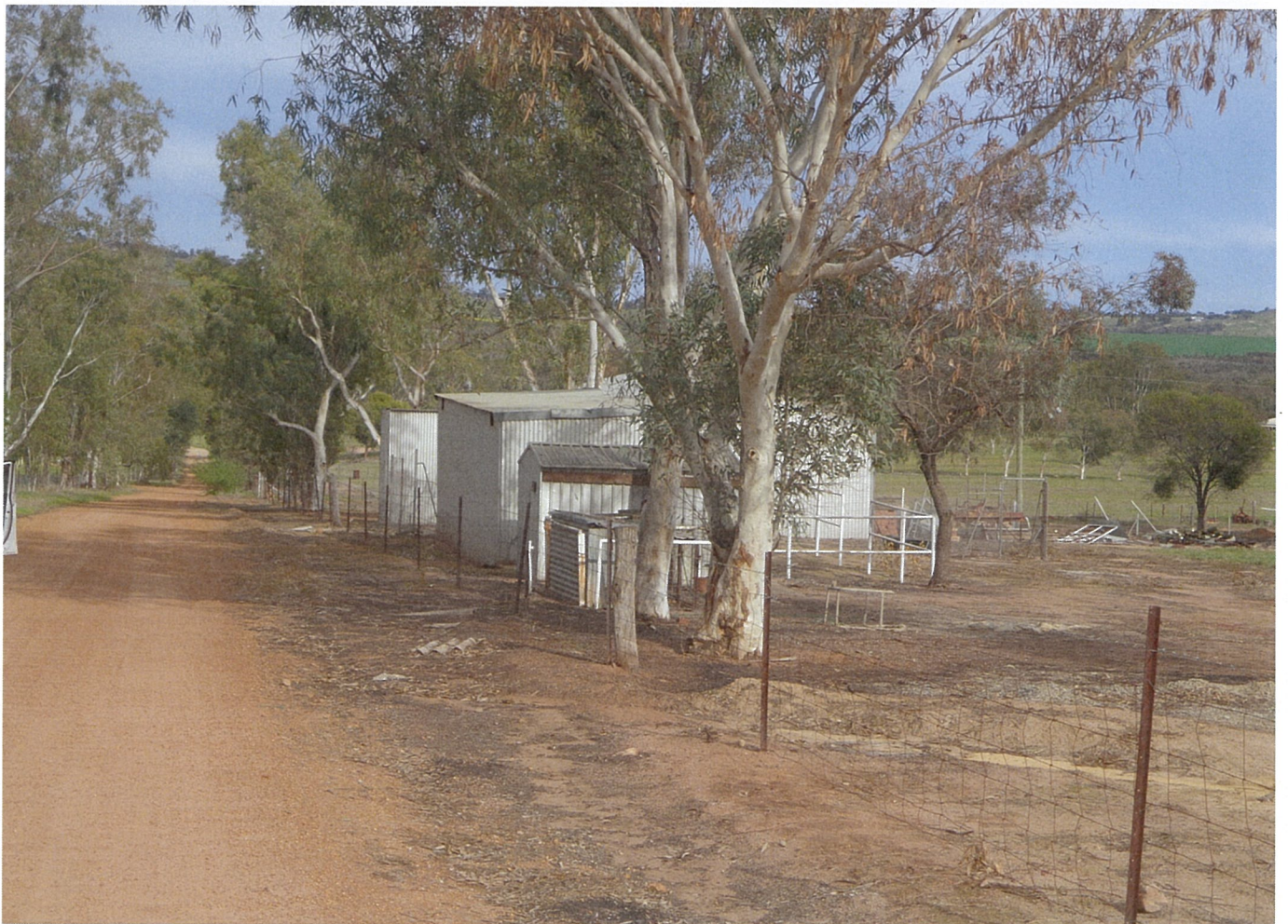
Photo 5: Stables & Sheds location in relation to boundary
