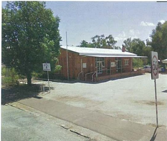
Plate 1. Looking NE across Subject site with existing RSL building in view
