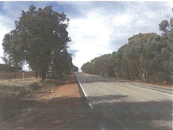
Plate 3. Entering sight distance looking east
