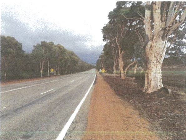
Plate 5. Highway approach to intersection from the East
