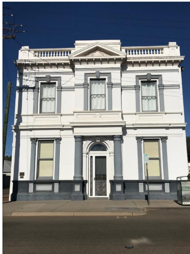
Street View: After Screen Door installed
