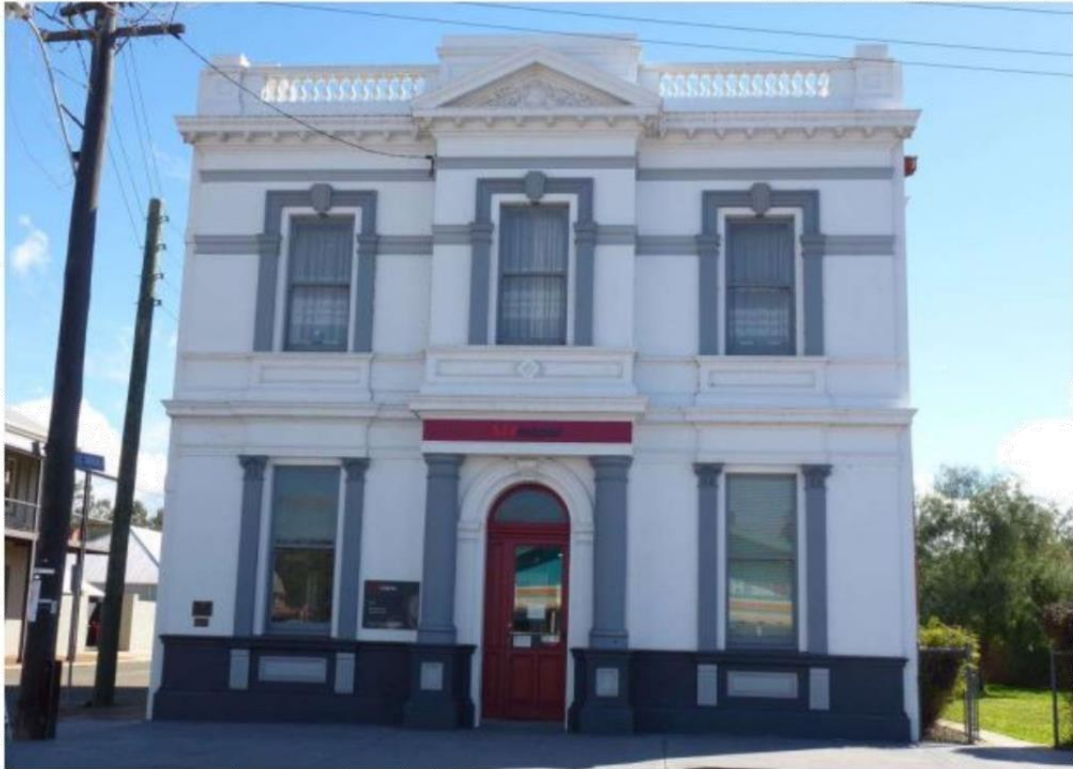
Street View: Prior to Screen Door being installed
