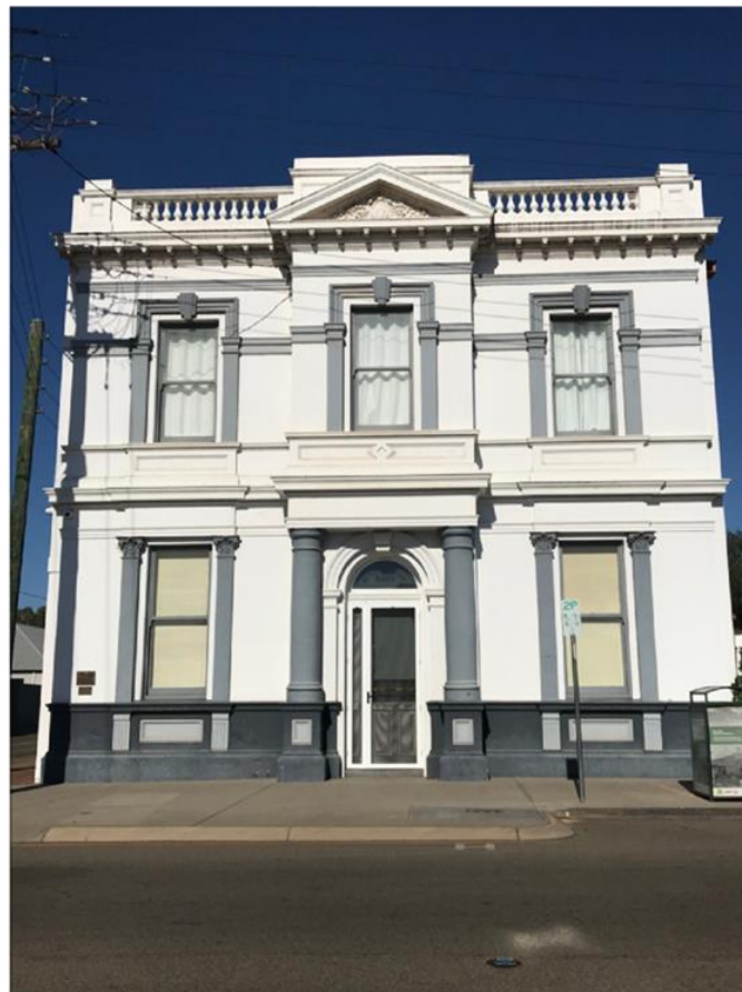
Street View: After Screen Door installed
