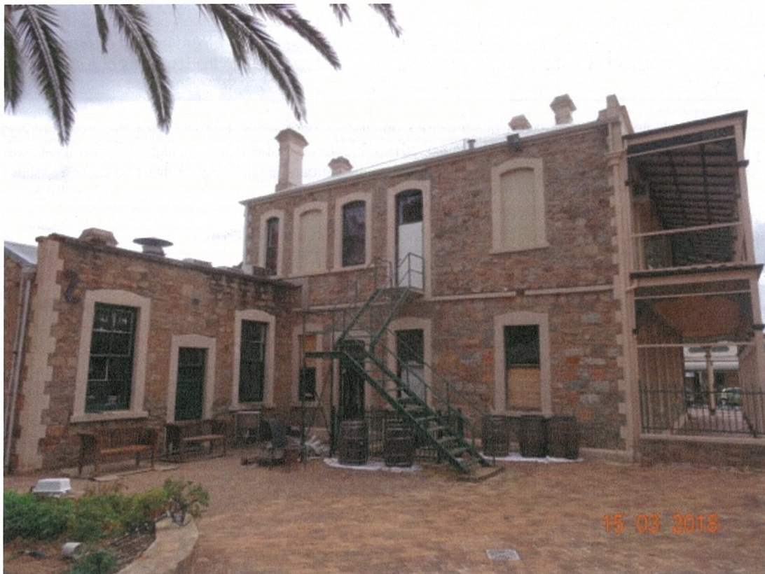
Figure 4 – Western elevation of the Imperial Hotel with the kitchen extension to the left and fire escape stairs which are being upgraded to meet BCA requirements. (Source: TPG, 2018).
