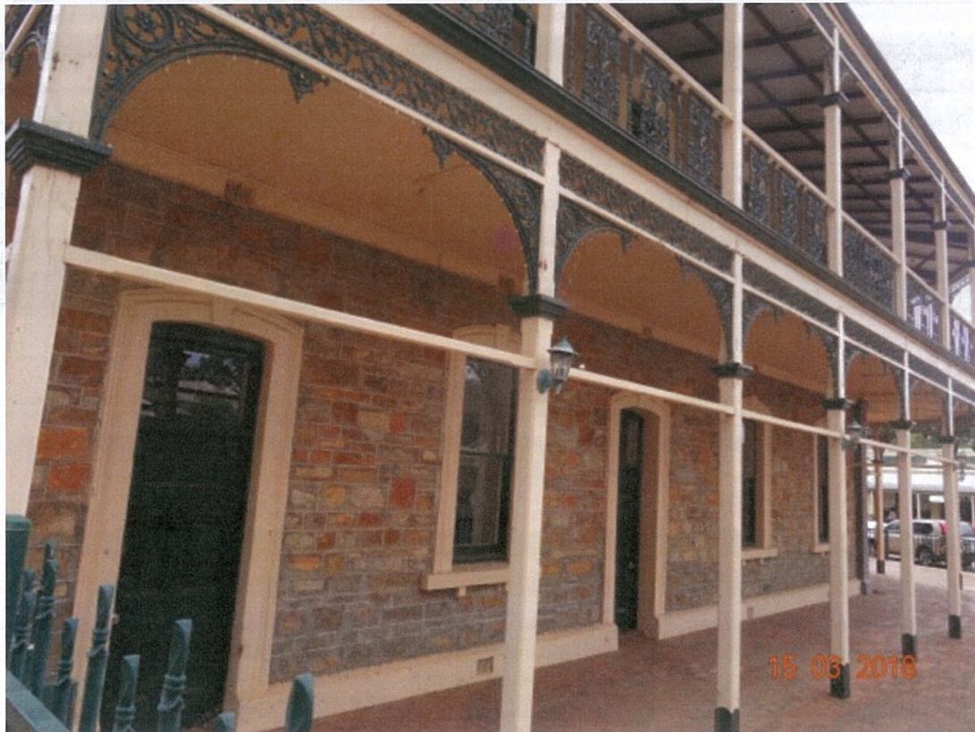
Figure 3 – Southern elevation of the Imperial Hotel where new café alfresco will be located. NB cement pointing to be raked out and replaced with lime mortar to match original (Source: TPG, 2018).
