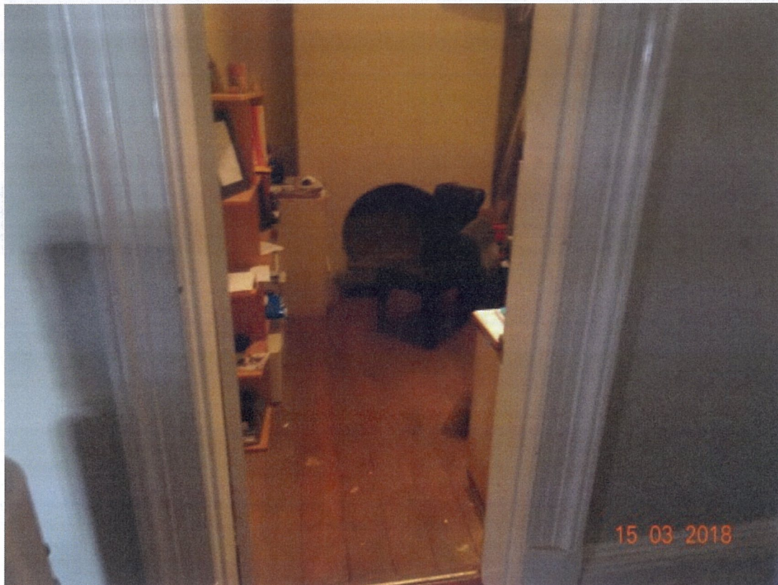
Figure 8 – View of the ground floor office being converted to accommodate a DDA accessible toilet. This door is being widened approximately 250mm, and the architrave will be reinstated. (Source: TPG, 2018).
