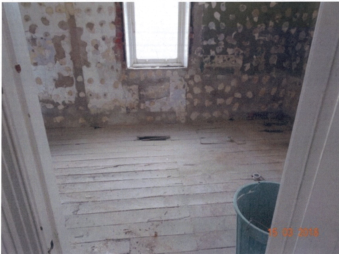
Figure 9 – View of former ablutions to the first floor with water damage to the timber floor and plaster being removed from the wall. This room will be returned to a bathroom use. (Source: TPG, 2018).
