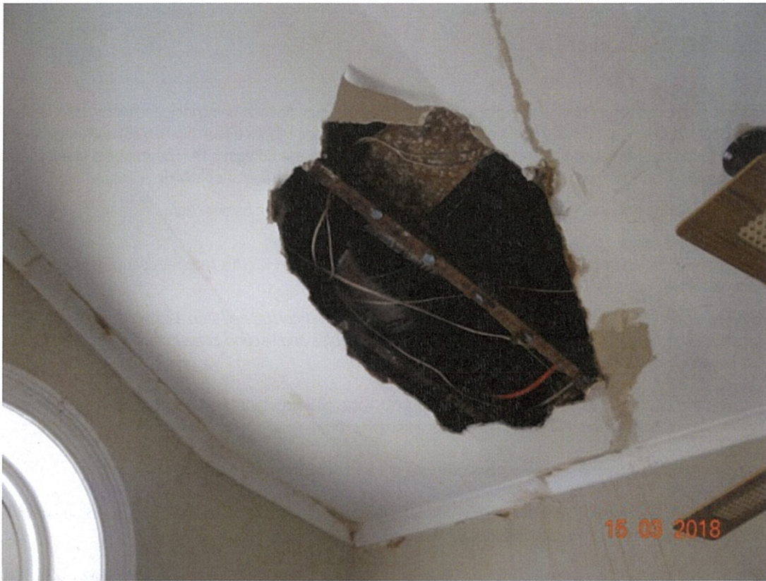
Figure 10 – Damaged plaster board ceiling panel to be repaired. (Source: TPG, 2018).
