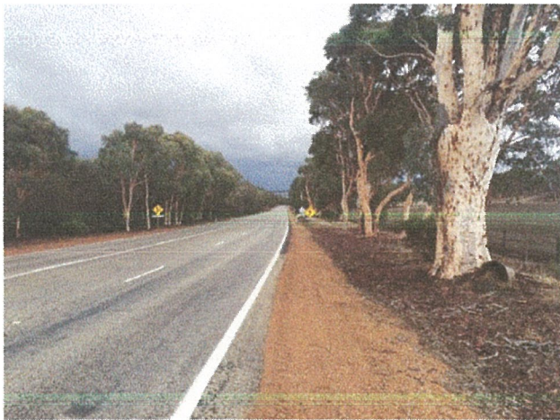
Plate 5. Highway approach to intersection from the East
