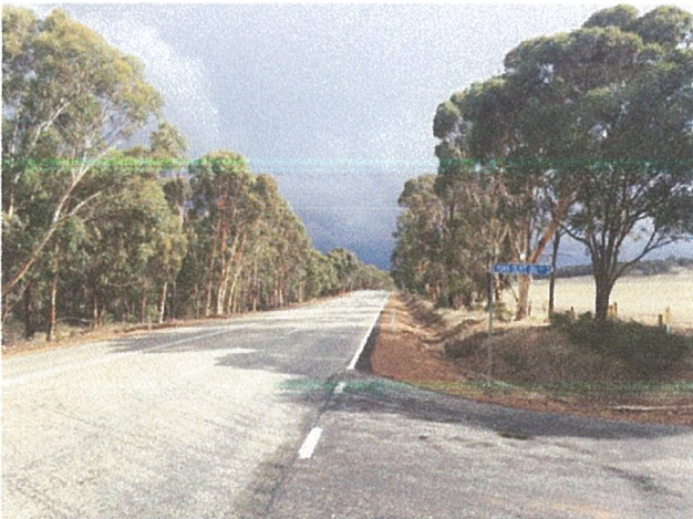
Plate 2. Entering sight distance looking west
