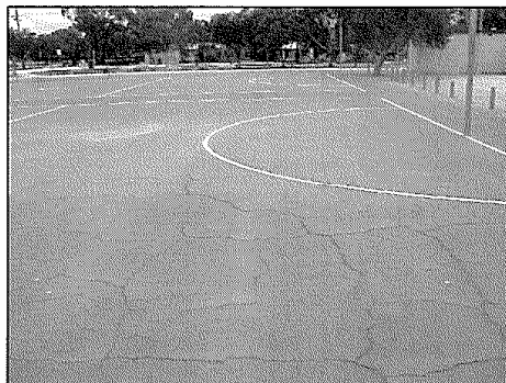
Heavily cracked surface
